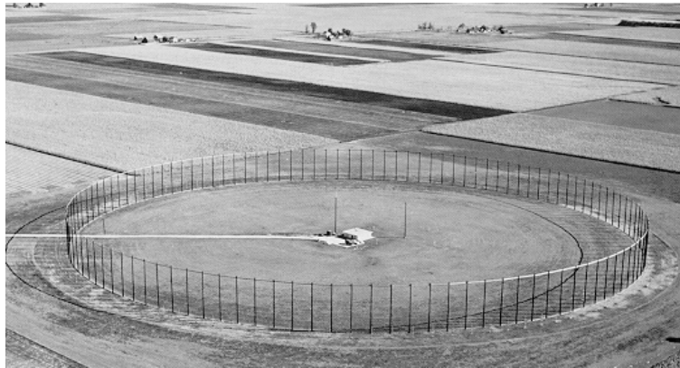
Figure 1.8: A large-aperture radio direction finding system known as a Wullenweber array at the Bondville Road Field Station, October 1960.
